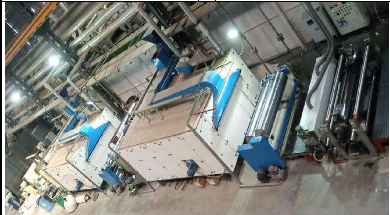
Printing Plant and Corona Treatment Plant Location in plant: Main Plant Use: For print different textures on the product, followed by corona treatment.
