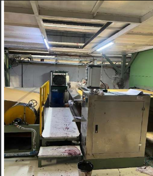
Machinery name: Foam Head Location in plant: Main Plant Use: Boiler to Provide Steam
